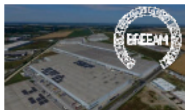
CTPBUCHAREST WEST PARK - BUW 16 DEPOZIT LOGISTIC
